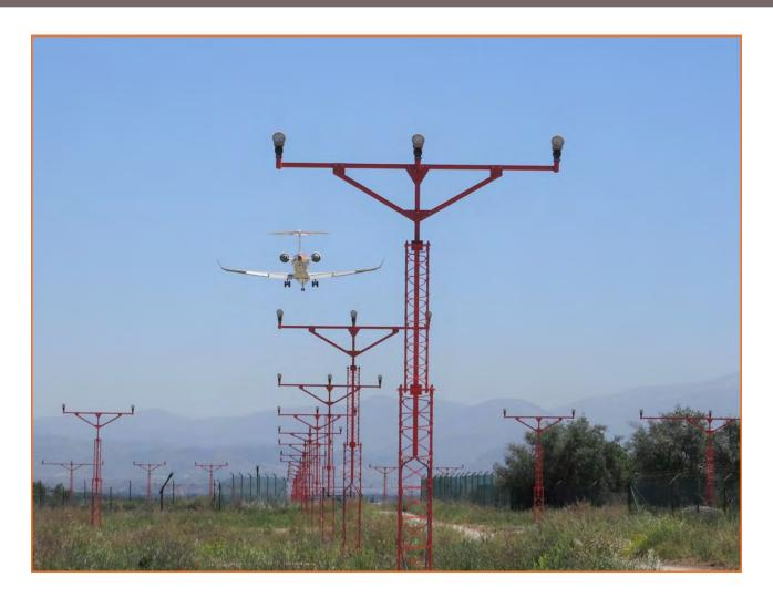
Millard Towers Approach Lighting System (ALS) masts are used to rigidly support equipment, yet yield if accidentally impacted. Frangibility has been confirmed by third-party full-scale impact testing and FEA modelling. In fact, Millard masts are present in ICAO Doc 9157 as examples of proper frangible design and testing.
