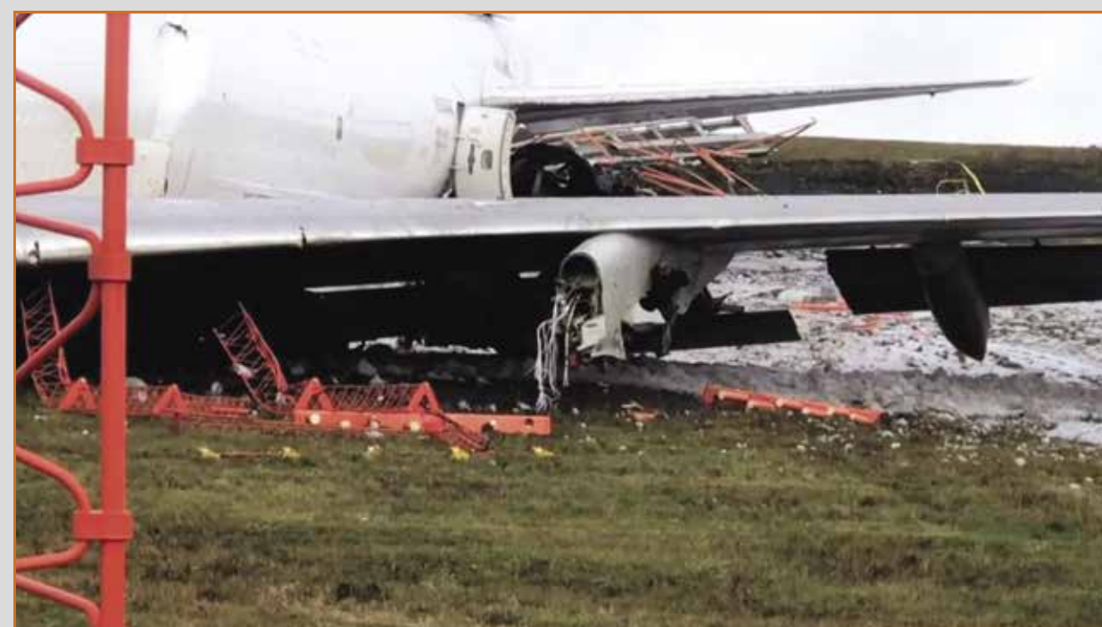
Millard Approach Light masts lay broken after being impacted during an overshoot approach.
