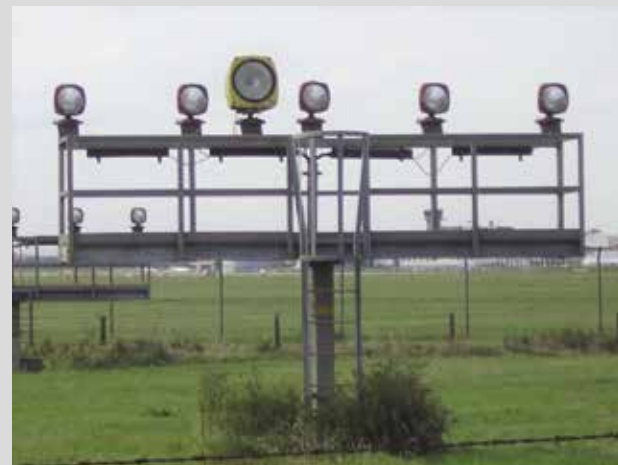
Traditional Non-Frangible Approach Light Mast
